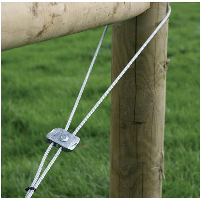
GPAK 6 - Installed as an H-Post brace
